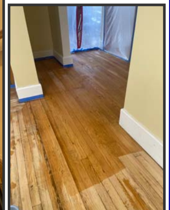
Results of our two Saturdays of working . . . steps and 2 rooms sanded . . . Picture on the left shows what the floors will look like after applying polyurethane
